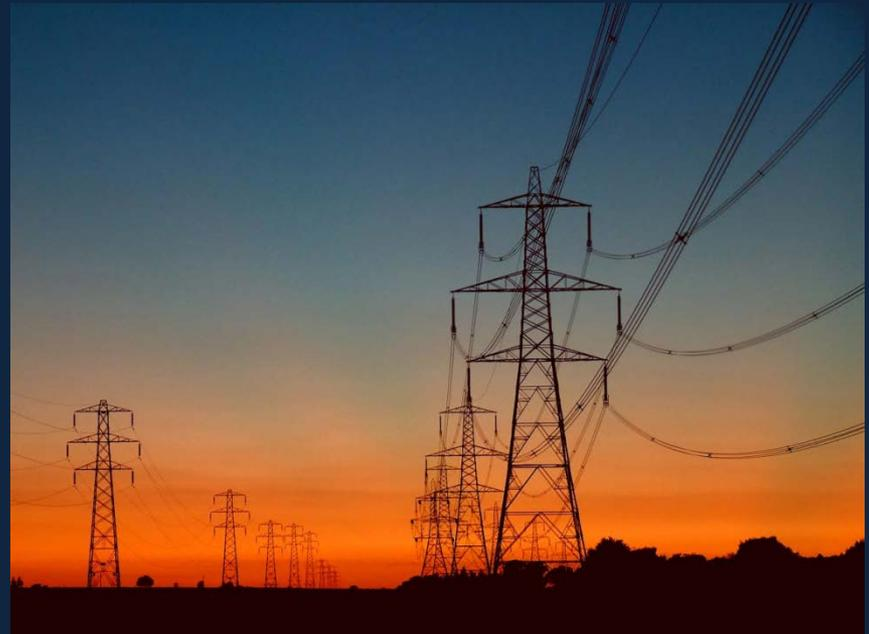
The power is carried by aluminum wires, suspended by glass, polymer, or porcelain insulators.
