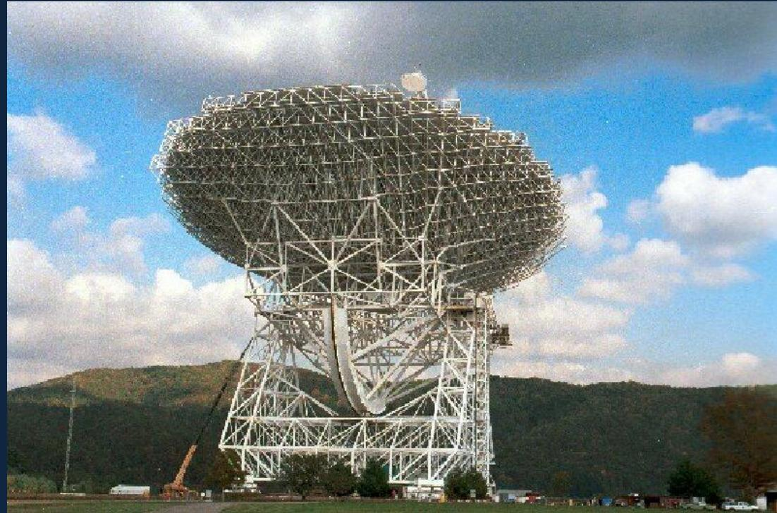
The receiver has diameter about 100m. Radio waves of wavelengths from 30 cm down are studied. Angular resolution around  $0.15^\circ$ .
