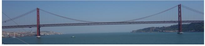
(Notice the vertical ropes are uniformly spaced horizontally.)
